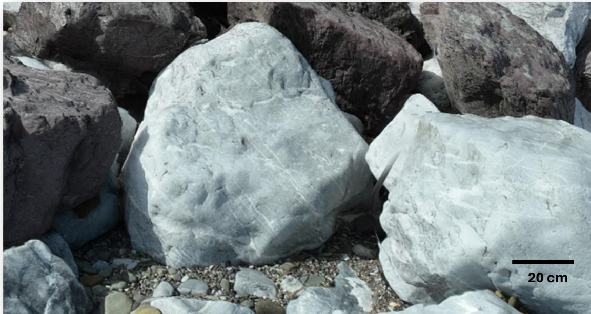
Figure 6. The image shows a portion of the coastal protection 3D model. Low-altitude manual drone flights were used to acquire imagery of features, allowing display of fine details in the rocks, such as the quartz veins in the limestone.
